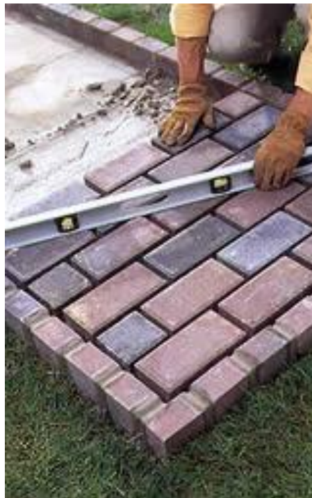
Figure 7. Laying in a cement mixture
