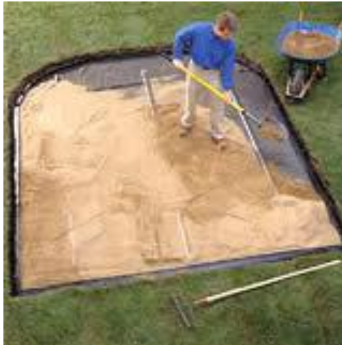
Figure 4. Geotextile laying between layers of fine stone and sand
