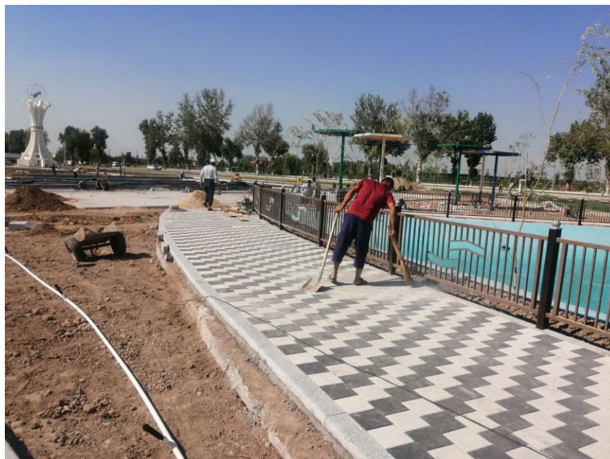
Figure 6. The final stage of laying pavement tiles
